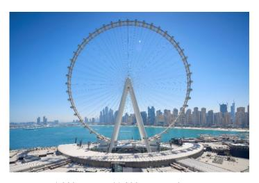
two hubs alone is 40m long, 20m high and weighs over 1,800 tonnes. 11,200 tonnes of steel were used in its construction – one-third more than the quantity used to build the Eiffel Tower. Ain Dubai has 48 cabins for which have the capacity to host 1,750 visitors simultaneously.
