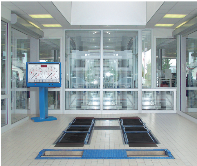
Workshop with flush-floor installed roller brake tester IW 2 LON ALL-WHEEL.
