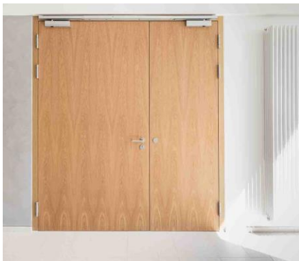
Left: double-leaf hold-open system as the third access to the council chamber Right: escape door to the outside with door closer and push bar
