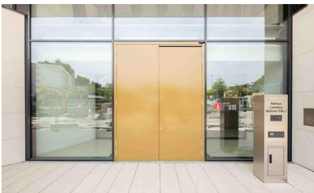
Barrier-free: the main entrance featuring automatic swing door systems with "robust" Powerturn drives
