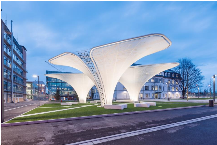
Three technically optimised OPV Solar Trees now stand in the redesigned entrance area of Merck KGaA in Darmstadt. (@Picture Merck KGaA)
