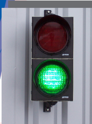
Ampelanlage | Traffic light
