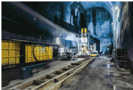
Photo 2: Nant de Drance, Switzerland
