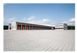
**Bild:** The new transhipment centre in Driedorf will be built in the shape of a Y. This concept has already proven itself at several other locations, for example in Herford (see photo). This means that more loading gates can be built on the same hall area than is possible with other designs.
