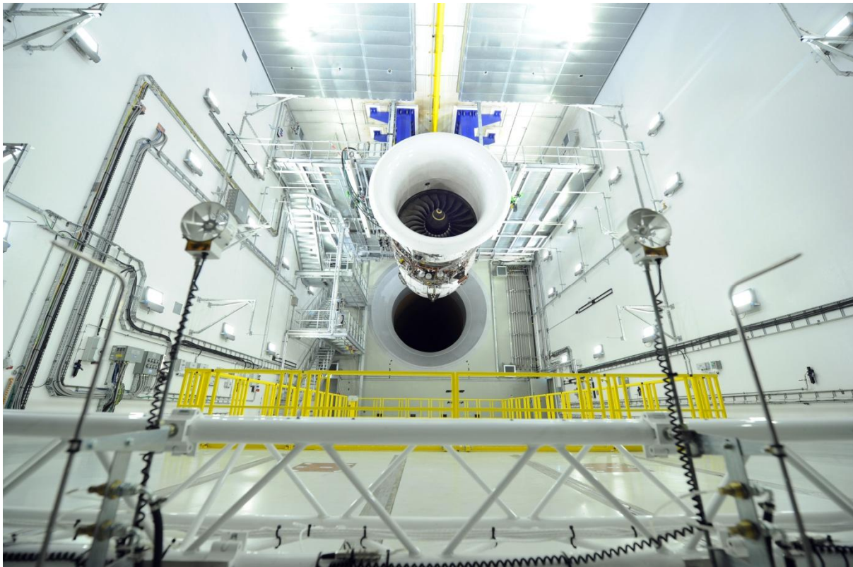
Fig. Nr. 10: View inside test cell with engine above the CTI Systems work platform
