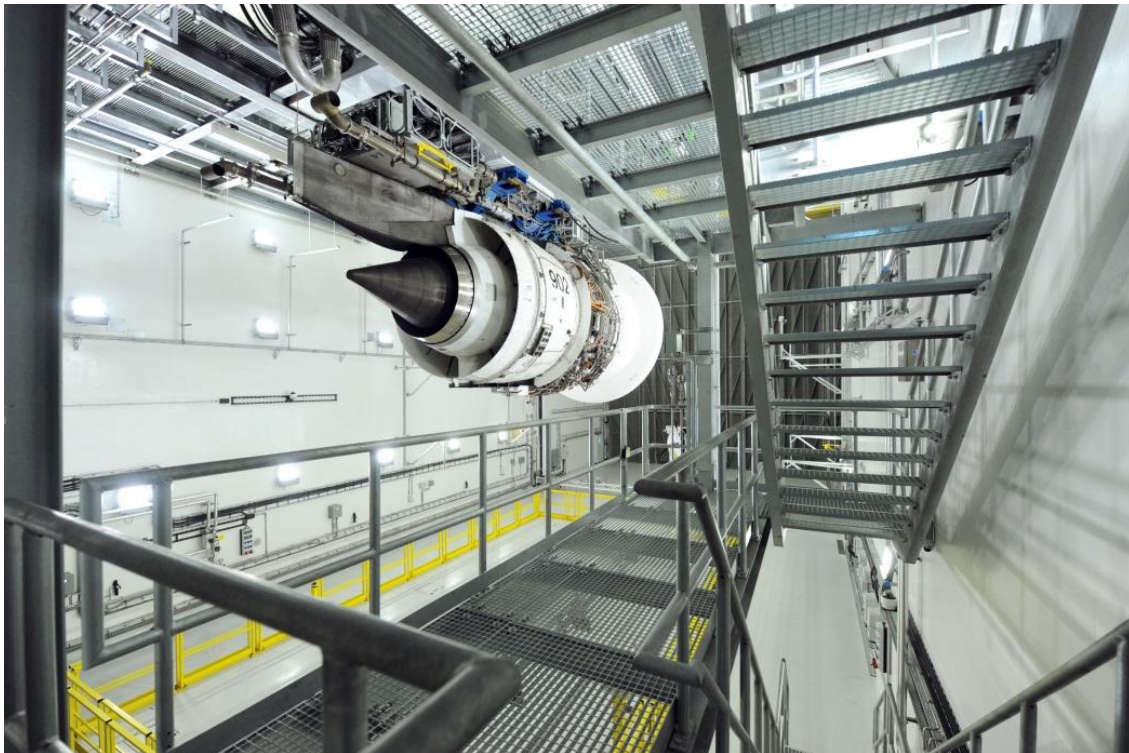
Fig. Nr. 6: Engine and maintenance platform inside test cell
