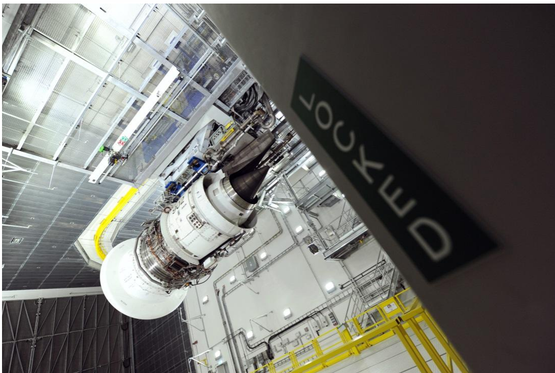
Fig. Nr. 9: Engine fixed on a Station inside test cell
