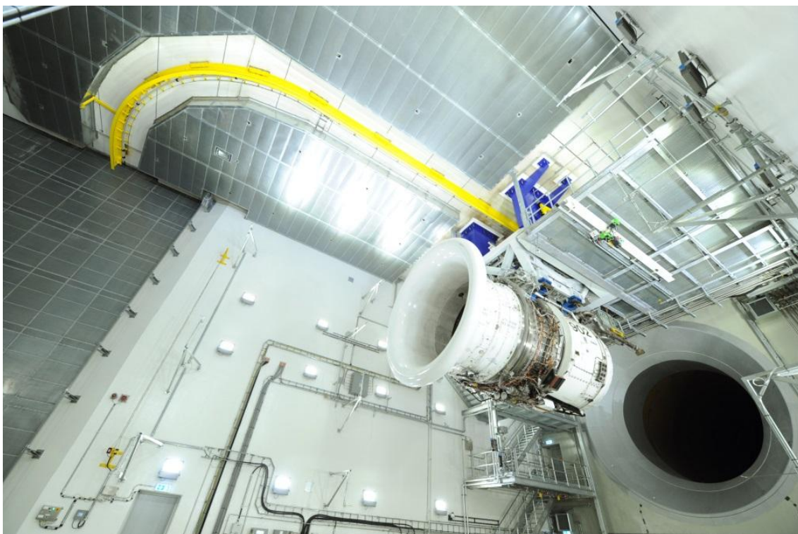
Fig. Nr. 7 & 8: Engine transport to test cell (closed test cell door on left side) and detail on Tarca rail interlock system
