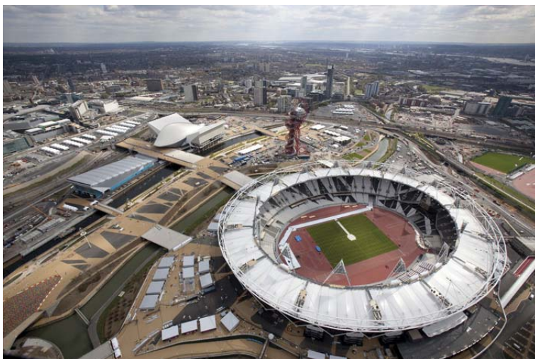
[Olympic Park, Copyright by LOCOG; GD_LOCOG_Stadium_4c_300dpi.tif]
