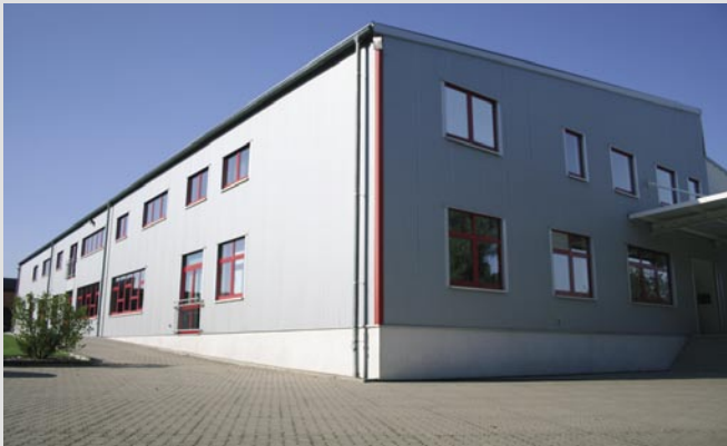
Production facility delpro
