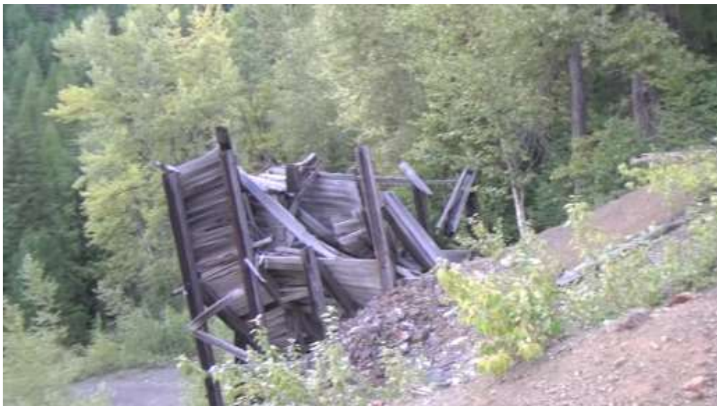
Photo of ore bin at former Protection-Goodenough mine.
