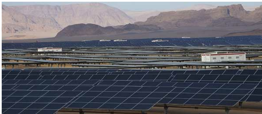
Image 2: 103 MWp Al-Quweira Solar Park near Aqaba, Jordan
