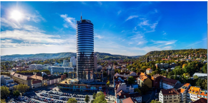
Jentower in Jena
