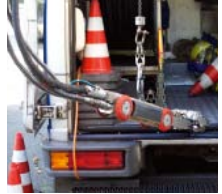
» High-tech in action. The Berlin water operations use remote controlled robots to inspect the narrowest channels.
