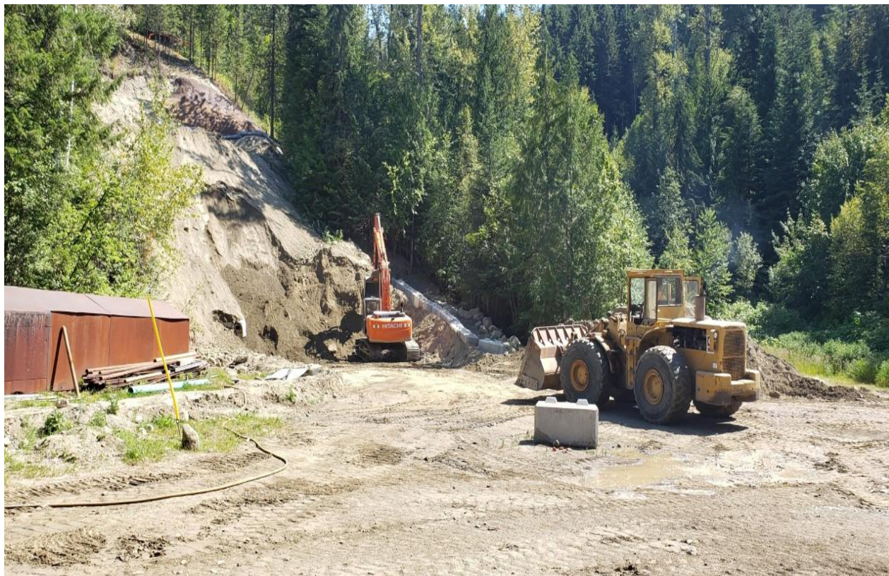
Photo of start of excavation using excavator and loader.
