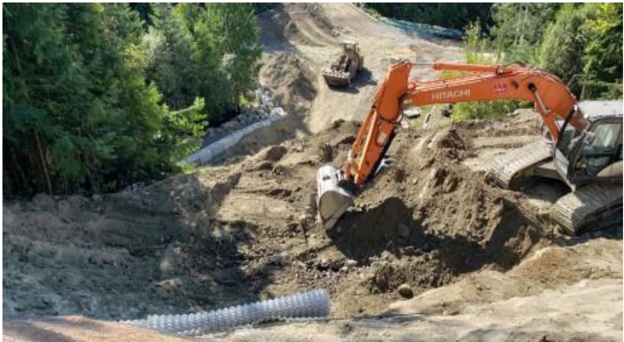
Photo of start of overburden excavation above portal height.
