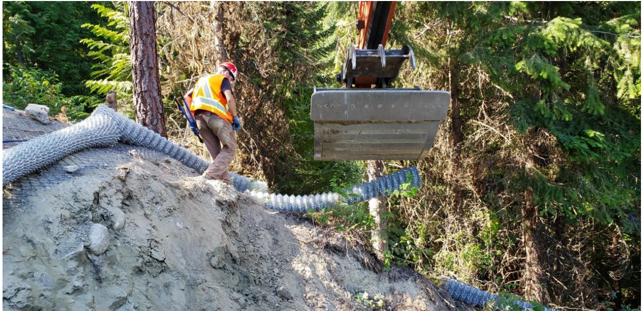
Photo of new screening being placed by Hitachi 180 excavator
