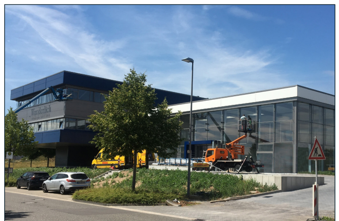
The final touch - the new Wunderlich company headquarters is almost complete and ready to move in
