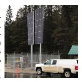
solutions are used to provide clean, reliable power for LED lighting at roadside brake check and chain off areas along the Trans-Canada Highway in Canada's Yoho National Park.
