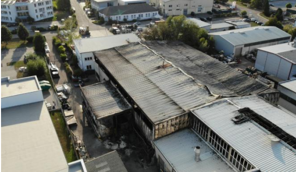
After the fire (Photo by HERBOLD)
