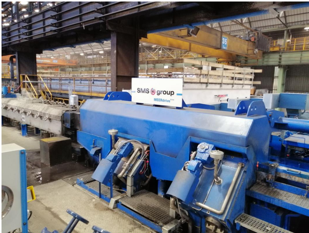
The SMS group MEERdrive ®PLUS sizing block in operation at ARLENICO works.
