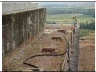
The hydrophilic limestone and inadequate drainage led to the soaking of the sub-structure. The affected retaining walls and cross vaults had to be lined with brick and protected against further water infiltration.
