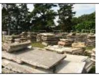
After successfully securing the stability, the up to two square metres big lime flagstones had to be newly fitted. At the same time, the sensitive lime flagstones are restored piece by piece.
