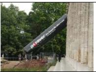
On two working days, the 30.06.08 and the 01.07.2008, a total of 150 m³ Poraver was gradually introduced. The expanded glass granulate was blown from the silo vehicles on to the site over a distance of 80 metres.
