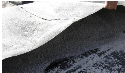
HDPE-barrier-chamber filled with Poraver File name: 31222 Beckenbau
