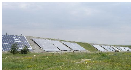
Solar cells are lined up on the exterior perimeter of the embankment to collect solar energy File name: 3121 Solarplatten
