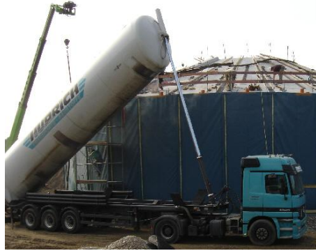
Preparatory work for the blowing-in of the insulation of the thermal energy storage silo in Munich. file name: : Wärmebeckenspeicher München
