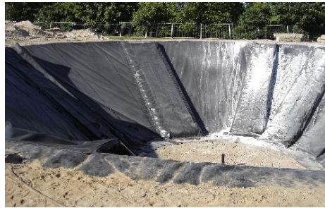
The insulator Poraver in HDPE barrier -chambers used to insulate underground thermal energy storage file name: 31222 Becken
