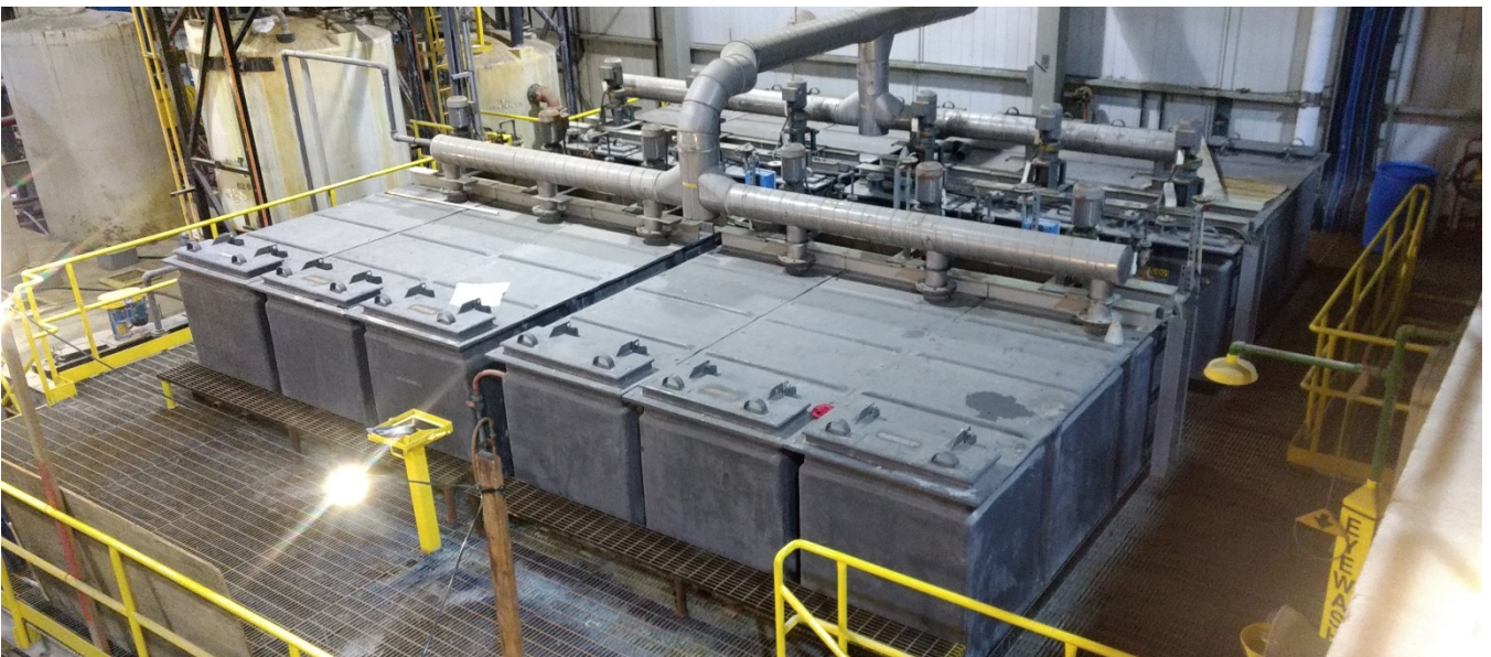
Power restored in the Solvent Extraction (SX) area
