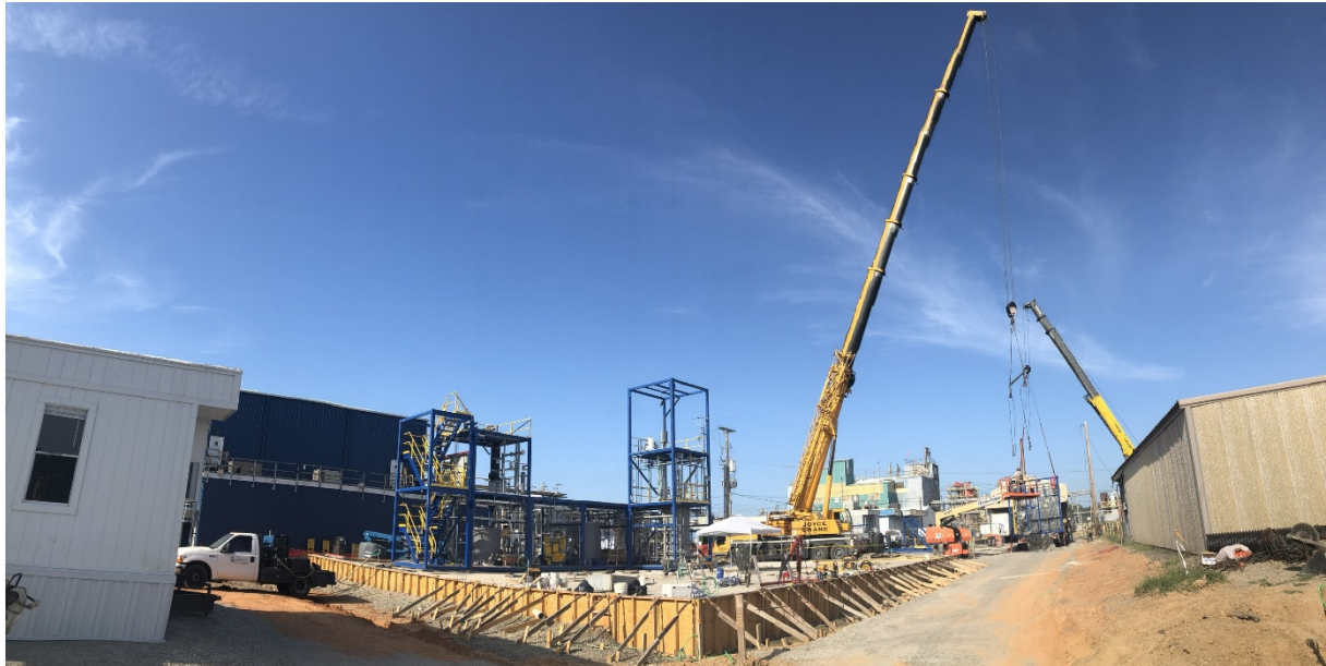
Figure 1. Building demonstration plant at Lanxess Project site
