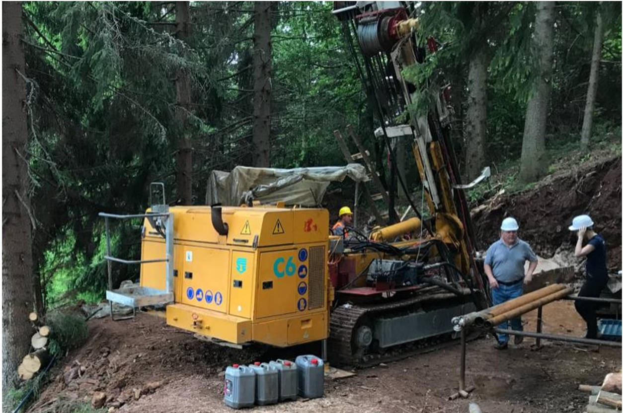
Drilling at Rupice
