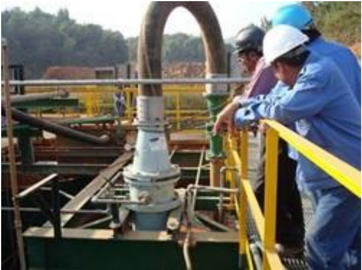
Figure 3: Aachen™ Installation - Gold Mine Example 1
