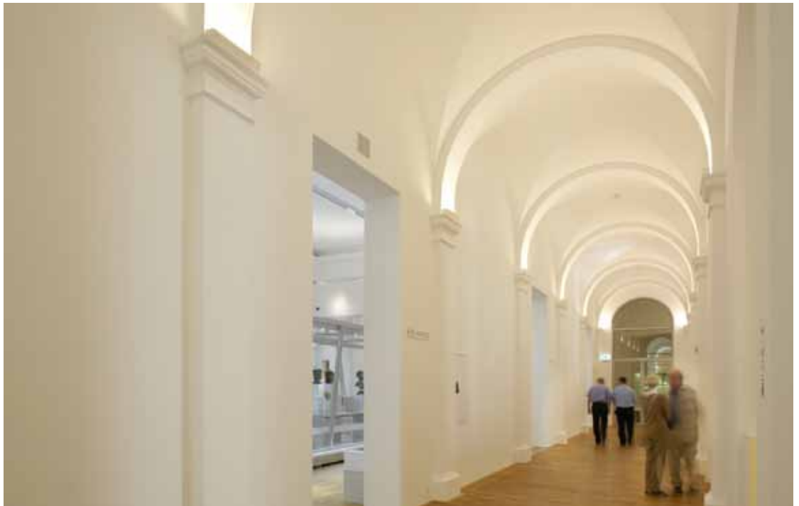
B2 | Discreetly built-in special luminaires provide attractive indirect illumination of the corridor ceilings.
