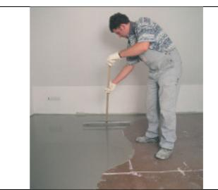
PCI Periplan Extra light is fiber reinforced, that flows easily and hardens quickly. Properties that pay off, particularly with renovation and upgrading work.
