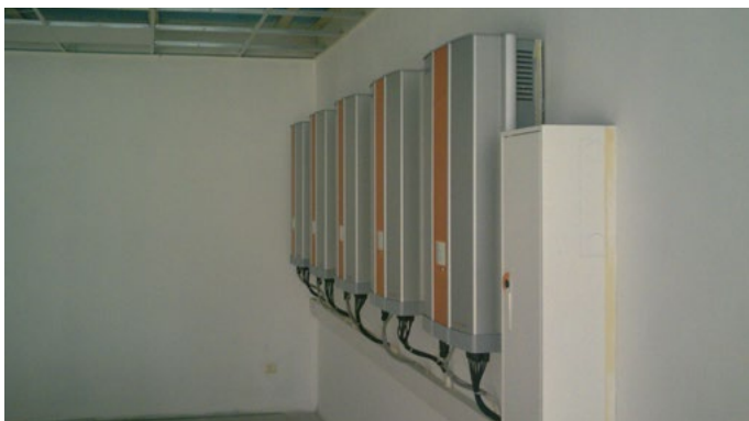
View of the SOLIVIA transformerless inverters installed in the K-W-H Energy GmbH office space.
