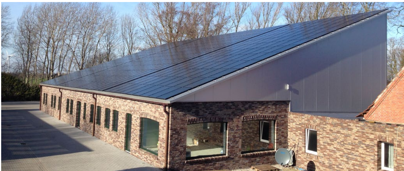
Photo: K-W-H Energy GmbH
