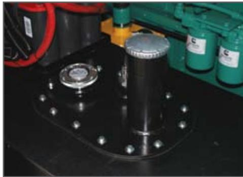
▲ **Mechanical fuel level reading placed next to the filling point**
