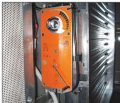
◀ **Automatic louvers with 230V antifreeze electrical resistance for easier opening at start-up of the generating set**
