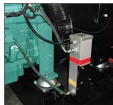
▲ Electric engine water heater
